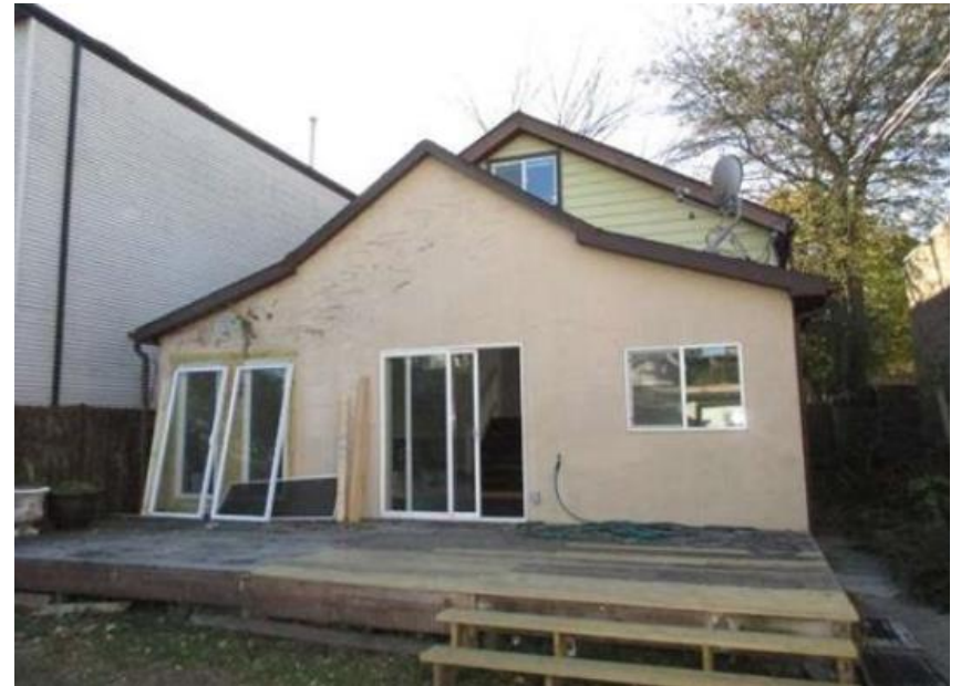
Rear view looking west
