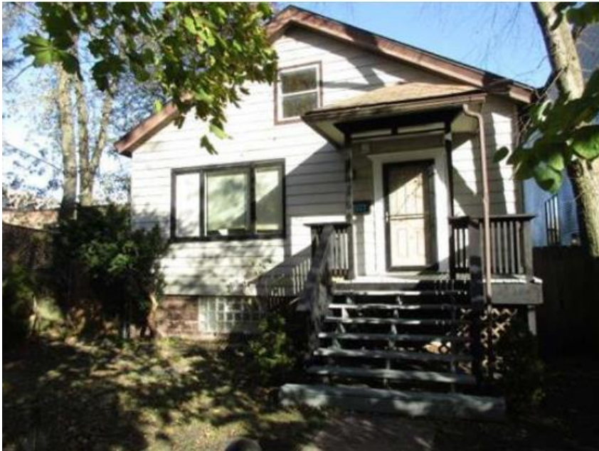
Front view looking east from Ravenswood
